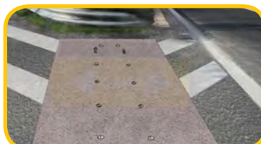
Base in cemento prefabbricata
