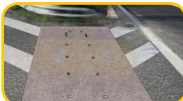
Base in cemento prefabbricata
